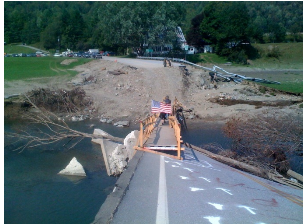
5 - Temporary footbridge over White River (Source: VTrans)
